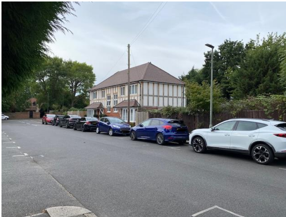
Figure 8 - Nos. 1A and 1B to the south
